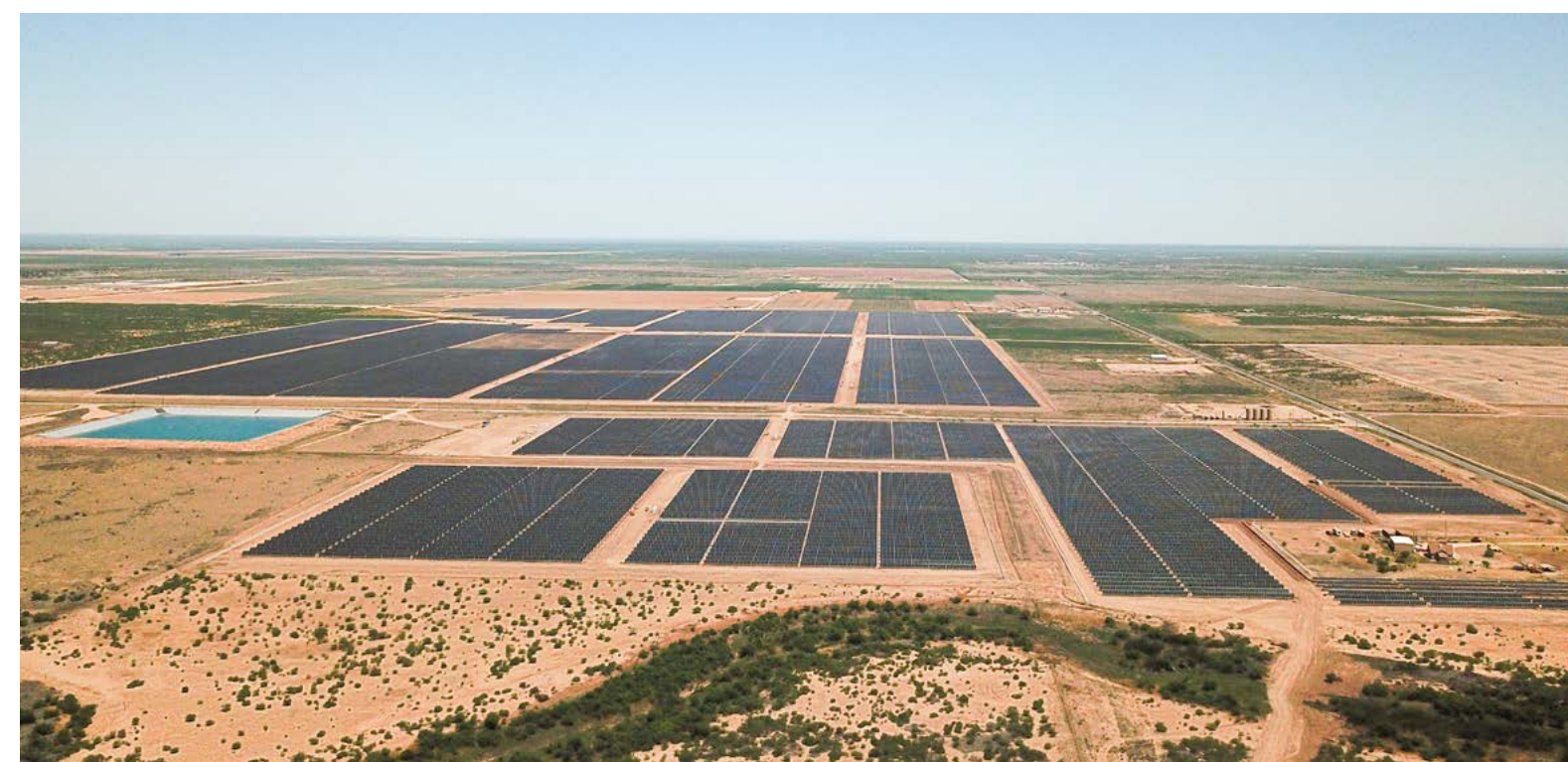
Nestlé’s large-scale solar energy investments will provide nearly half our electricity in the United States.
